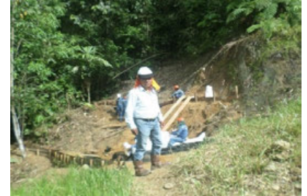
Local monitor in place
